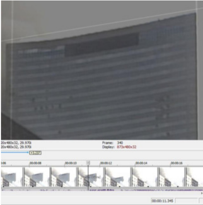
Figure 8 - At frame 340 ("2.0 s" at 11.345), significant vertical displacement is apparent along the entire north face, including both northwest and northeast corners. Global collapse is underway.
